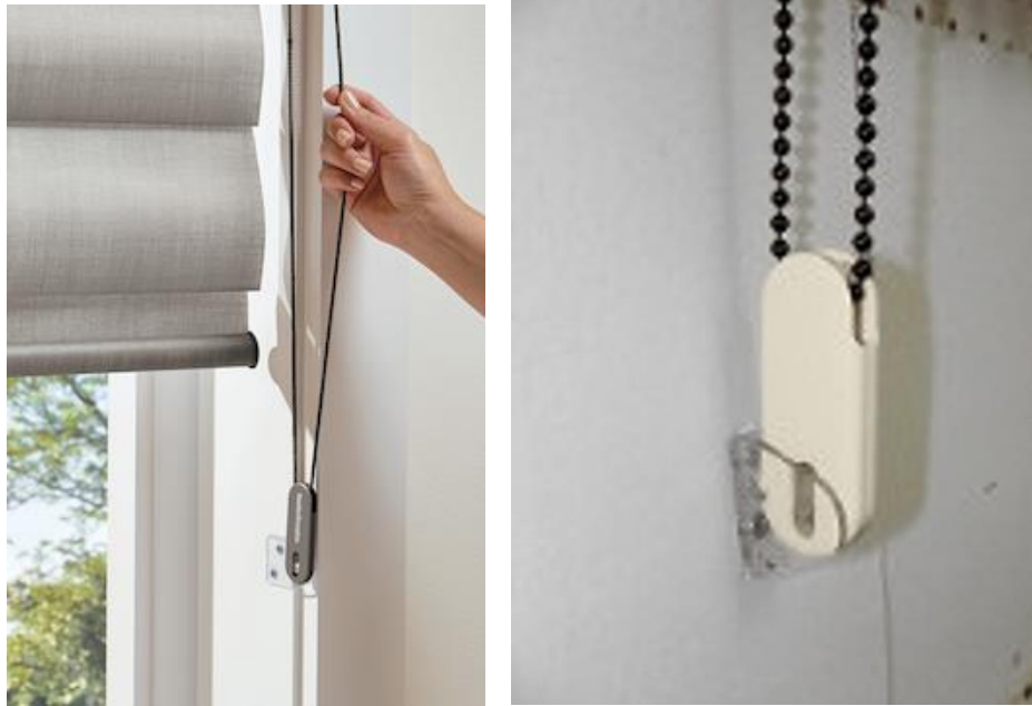
Figure 4. Typical installation of a tension device: 4(a) inside mount to jamb ( Secure-child-safe-cords-cord-tensioner-pirouette-Skyline-Window-Coverings.jpg (900x601) (skylinewindowcoverings.com) , 4(b) outside mount to wall ( Universal Cord Tension Device for Roman Shades 6 Colors DIY - Etsy ).
